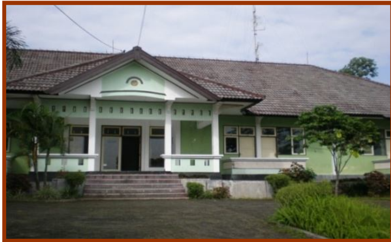
Gambar 9 Gedung Asrama B2P2VRP
